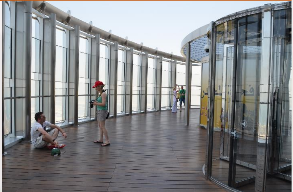
Outside viewing platform at the Burj Khalifa uses a steel framed glass barrier to prevent falls and offer protection from wind and wind blown sand
