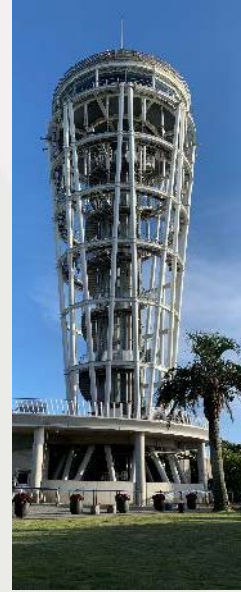
Enoshima Tower, Japan
